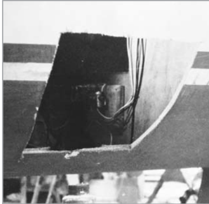
Figure 5-15 Remove the damaged section.
