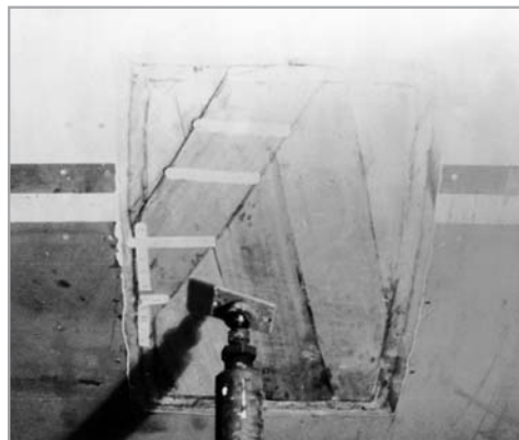
Figure 5-18 Bond the second layer in the opposite diagonal to the first layer.
