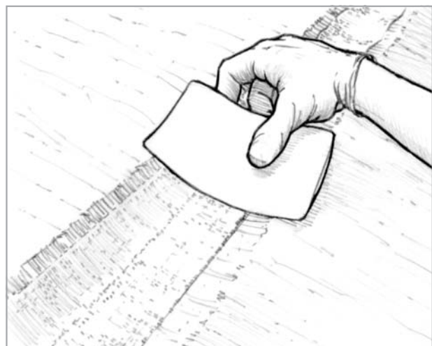
Figure 5-11 Apply fiberglass tape over the prepared joint.
